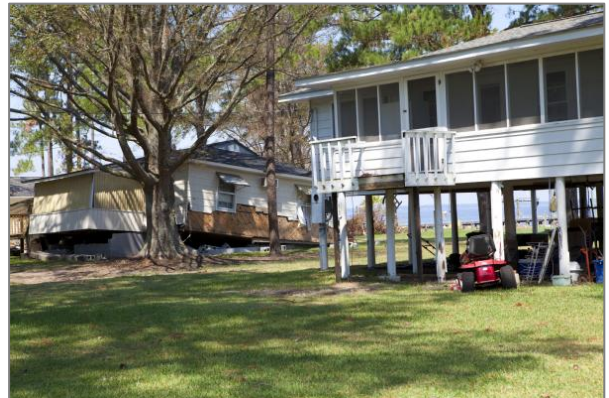
The elevated house on the right received only minor damage when Irene pushed 5 feet of storm surge ashore in North Carolina. The house on the left was completely destroyed.
