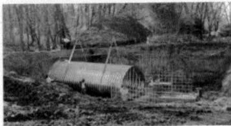
Crews install culvert that will go under new Cypress Lane footbridge.
